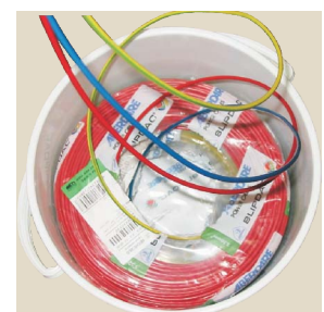
Photo 2: Extraction of 3 or 4 wires simultaneously from coils held
